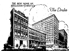
THE NEW HOME OF HELLESOE-STREIT CO. EAST WAGON 30-37 TELEPHONES SUPERIOR 4513, 4514
