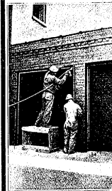
Spraying With Peerless Spray-Gun and Siphon Jar
