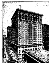
Edison Building Chicago, Illinois
