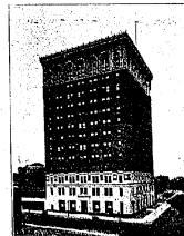
Nebraska Telephone Building Omaha, Nebraska
