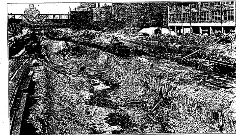
Union Station Project—Chicago
